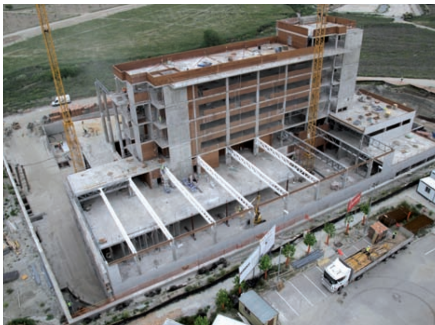
Figure 3. Construction of IMDEA Materials Institute
